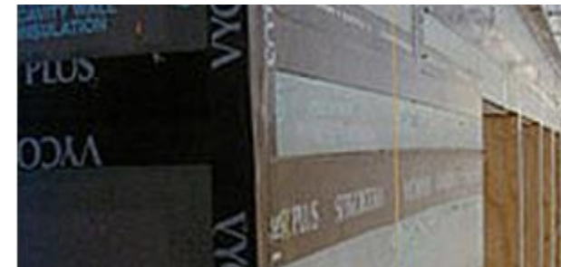
Sealed and Taped Boards or Building Wrap
