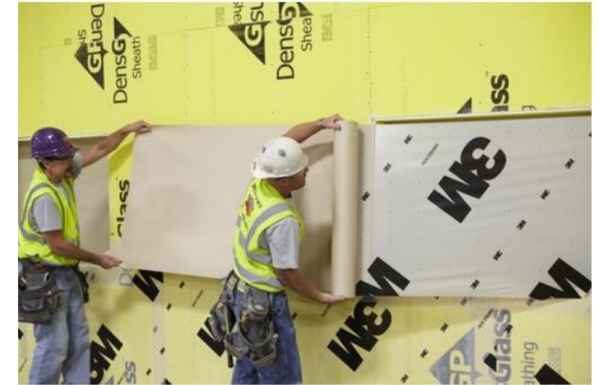
Sealed and Taped Boards or Building Wrap
