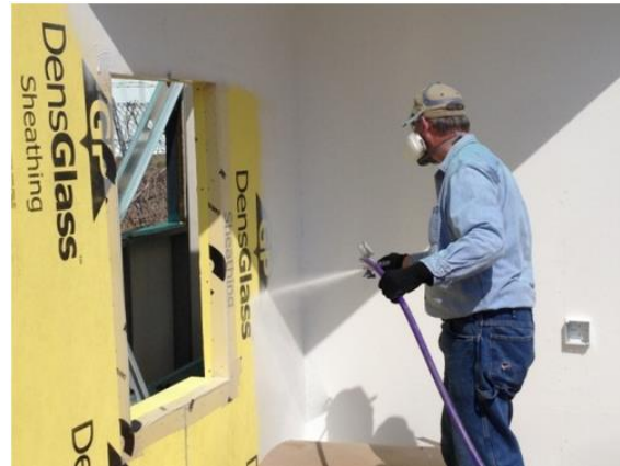
Sealed and Taped Boards or Building Wrap
