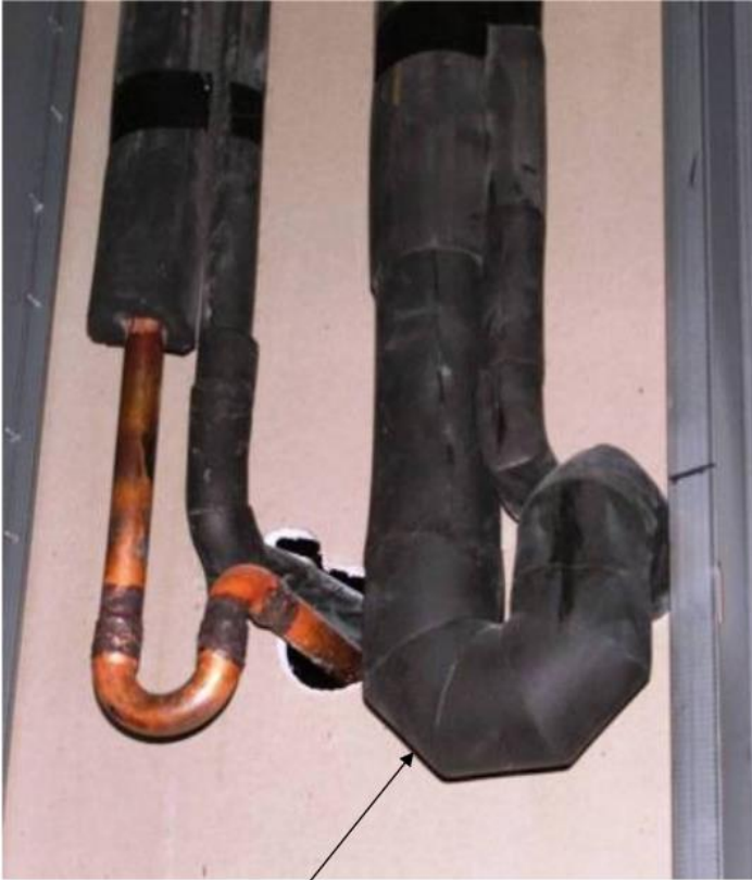
Mitered joints to prevent compression/stretching.
