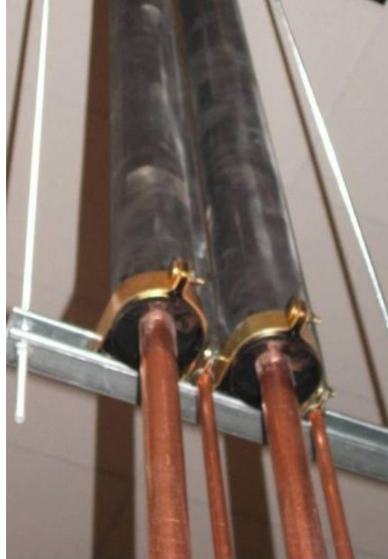
Hangers & supports enclose insulation – no compression
